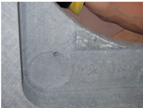
28. These two milled holes fit over the bracket just installed, holding the top panel in place.
